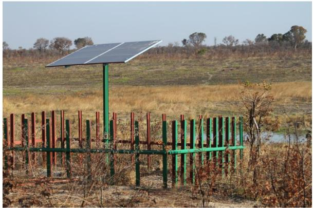
Figure 9. Tumbaeque waterhole in Bicuar National park. The solar panels to run the pump are visible in the foreground, with the waterhole and game trails visible in the background. In the interior of Bicuar park, only those waterholes that have pumps retain water year round.
